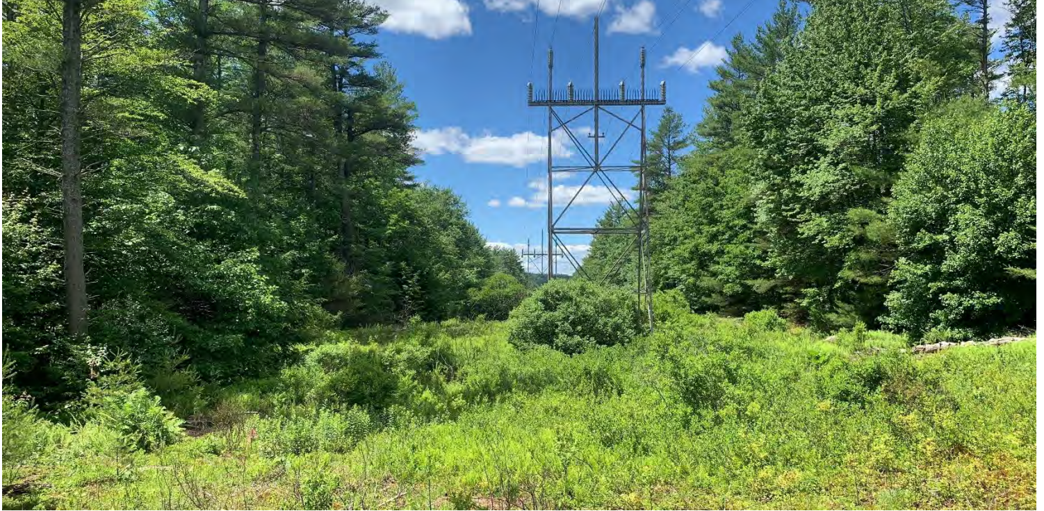
Photo #1: View of wetland GA-W5A near Str 414.
