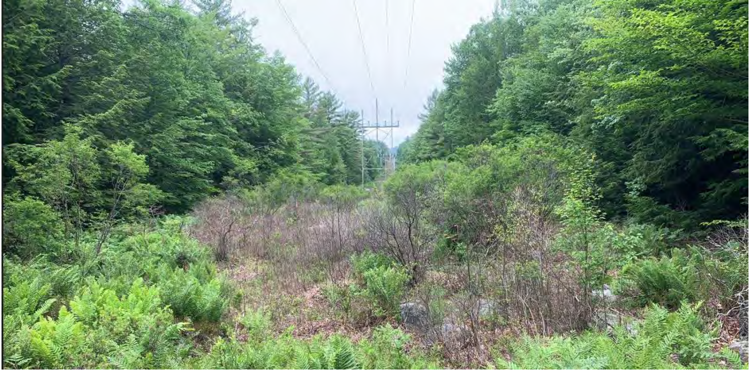
Photo #3: View of wetland RO-W6 looking at structure 205 in distance.
